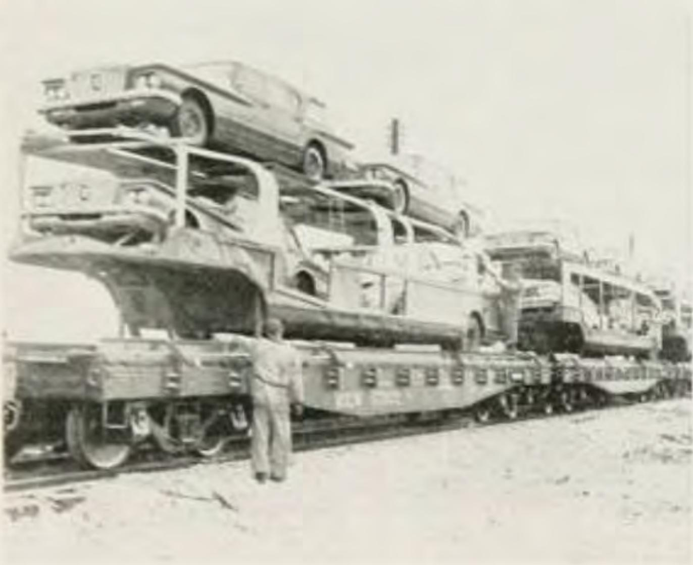
**Carrying multi-deck highway trailers likely led to the elimination of the trailer in favor of the multi-deck frame directly on a car – the Autorack.**
